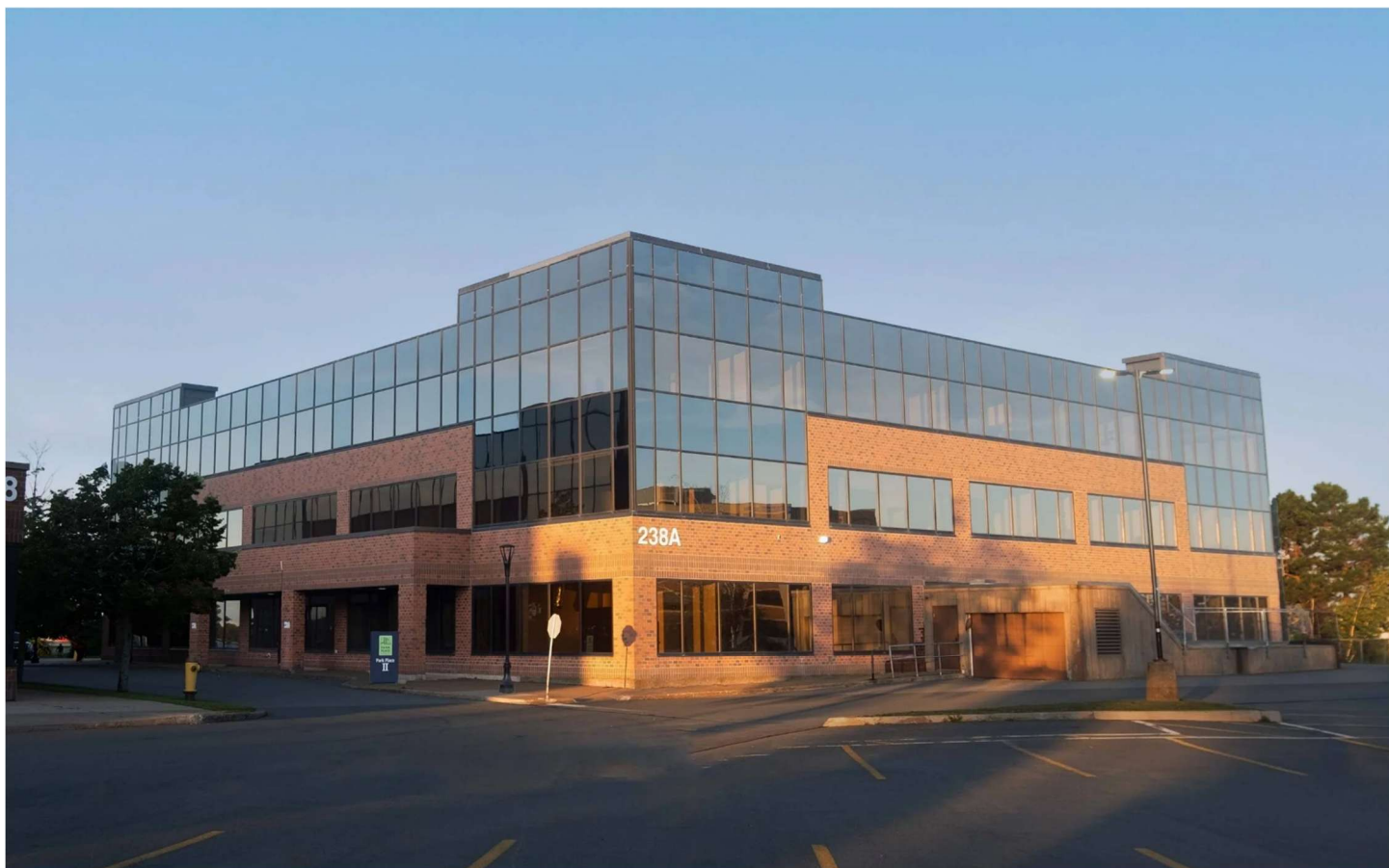
Photo: New AMI/CMDC Office, Modspace Unit 020 - 238A Brownlow Ave, Dartmouth, NS B3B 2B4
